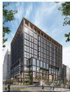
④ONE FUKUOKA BLDG.
